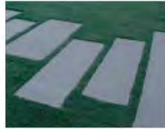
cip concrete slab walkway
