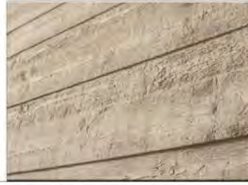
board form concrete
